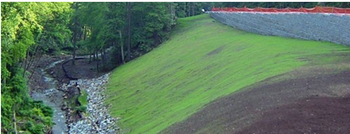
Seeded compost erosion control blanket, photo courtesy of Filtrexx
