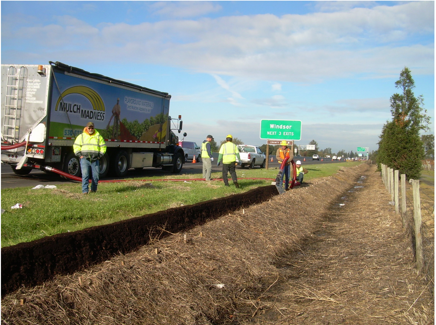
Compost Berm replaces multi-failed silt fence, Highway 101, Windsor, CA, photo courtesy of Salix Applied Earthcare
